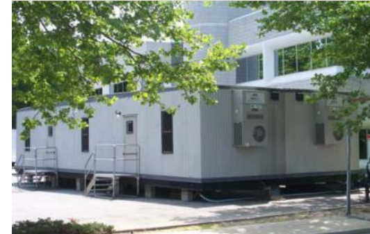
Mobile Office Solution
