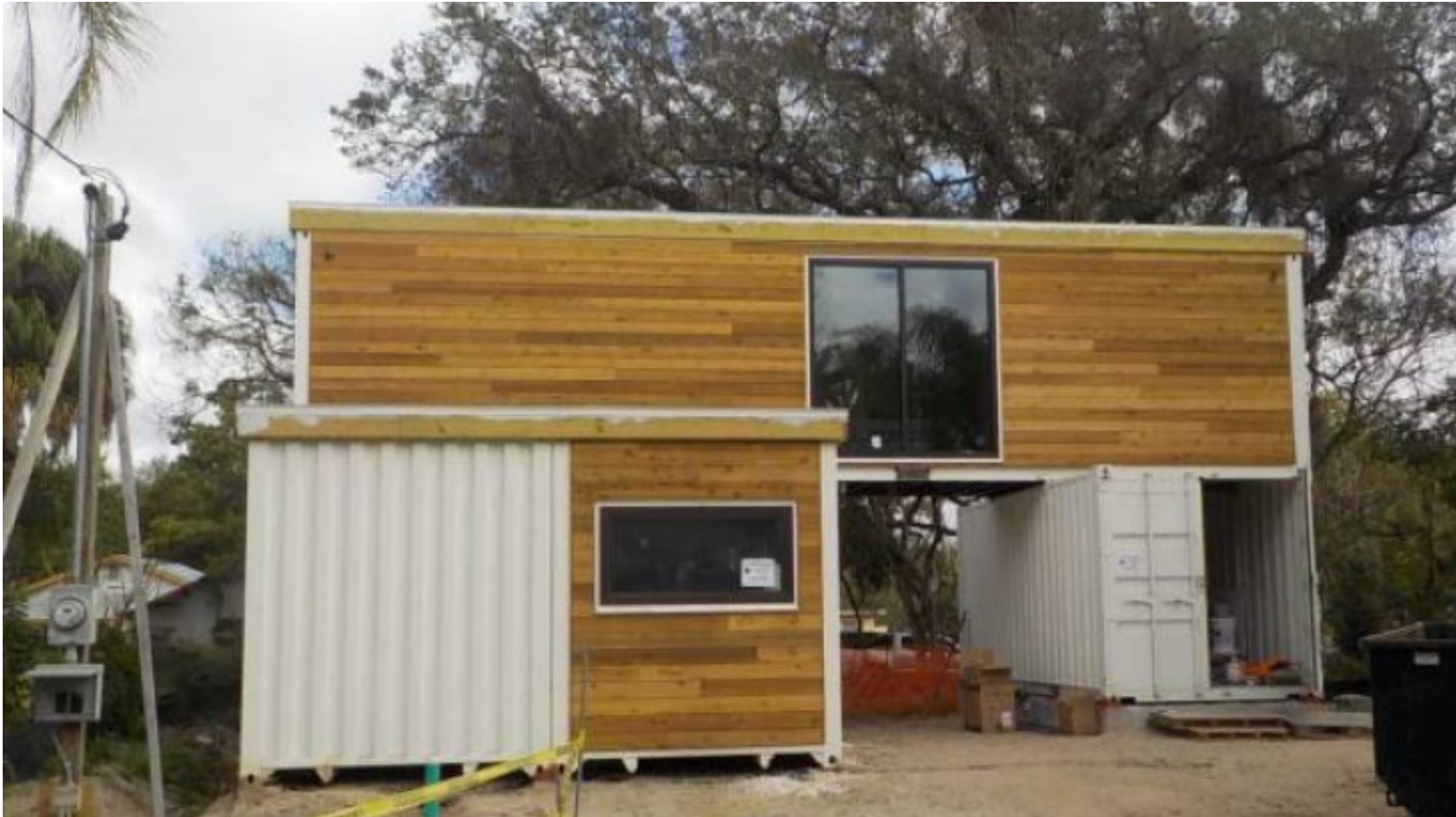
Home under construction in Tampa
